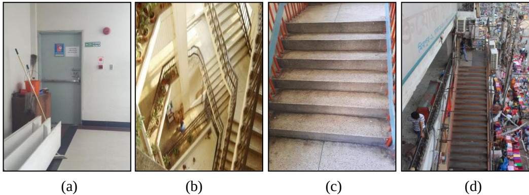
Fig. 3: (a) Locked emergency gate in Bashundhara City Shopping Mall, (b) Open stair will be a carrier of fire and smoke in Eastern Plaza, (c) Sloppy and narrow emergency stairs in Motalib Plaza and (d) Narrow and weak steel frame emergency stair in Muktijoddha Super Market
