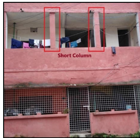
Photograph 1: Appearance of Heavy Overhang Photograph 2: Appearance of Short Column
