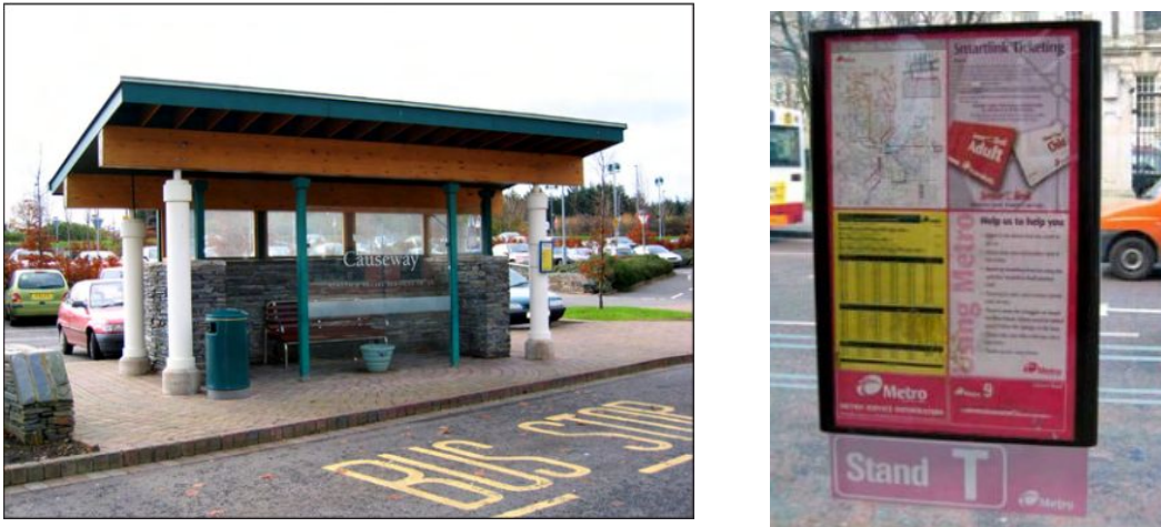
Figure 3: Bus Stop Facilities: Shelter and Information Board
