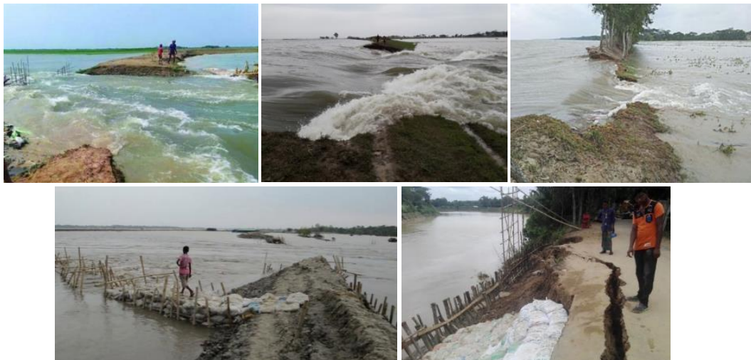
Figure 3. Embankment Breaching, Poor Construction, Operation and Maintenance
