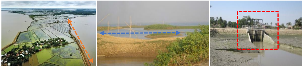
Figure 2. Embankment, Submersible Embankment and Polder
